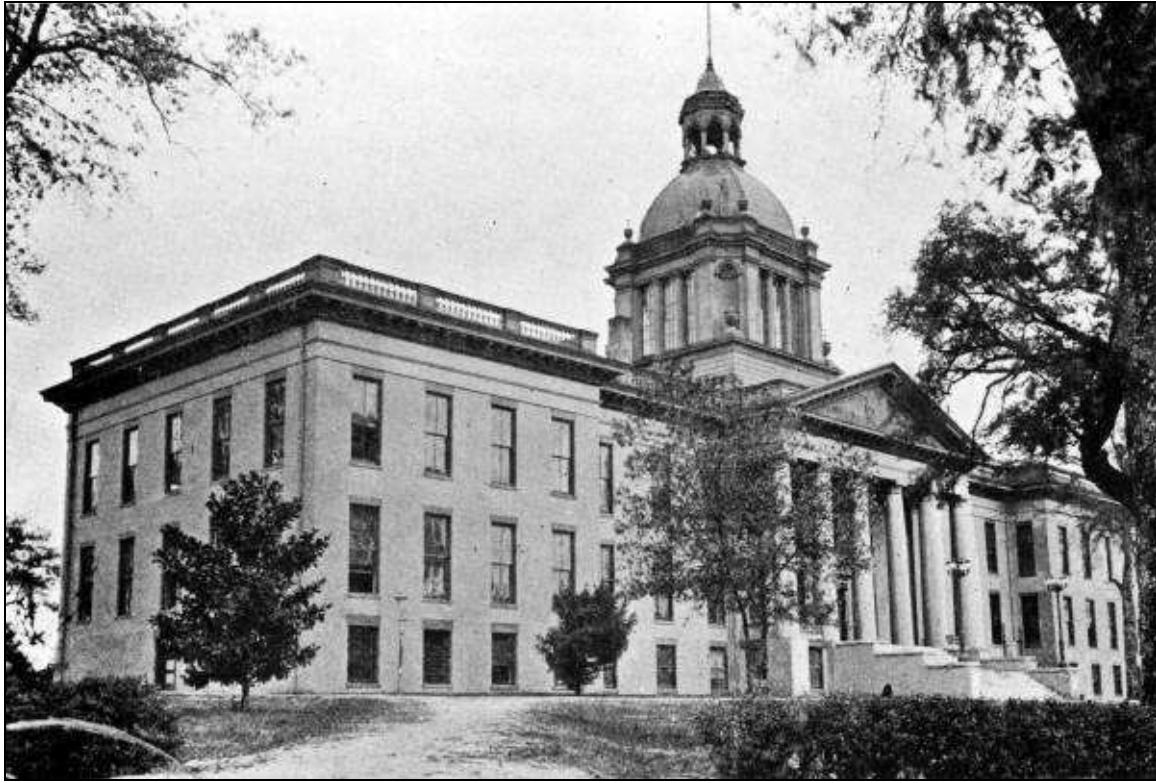
Remodeled Capitol, with new dome and wings (N and S)
